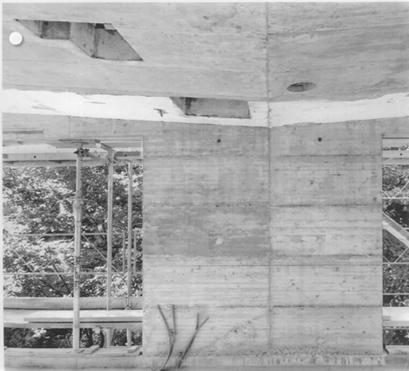
The load-bearing concrete construction with internal insulation takes up the facades and determines the appearance; short wall slabs and solid floor slabs, vertical and horizontal components, together create a repeating T-shaped motif. The floor slabs do not feature a separating joint at the thermal boundary and cantilever out. Local insulation inserts prevent the formation of condensate. (tl)
